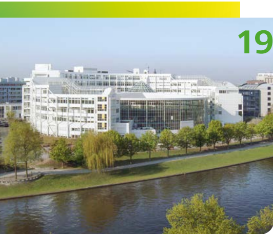
The award-winning Production Technology Center Berlin was inaugurated in 1985. Executive vice president of finances Hans-Ulrich Wiese began to equip the institutes with modern buildings and laboratories.
